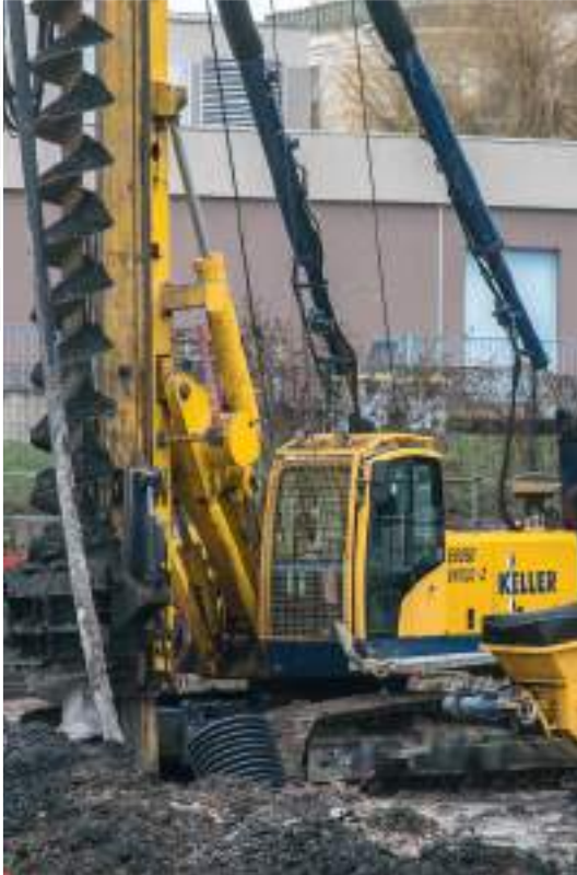
FRANCE E6050 LM – CFA240 CFA Piles.
