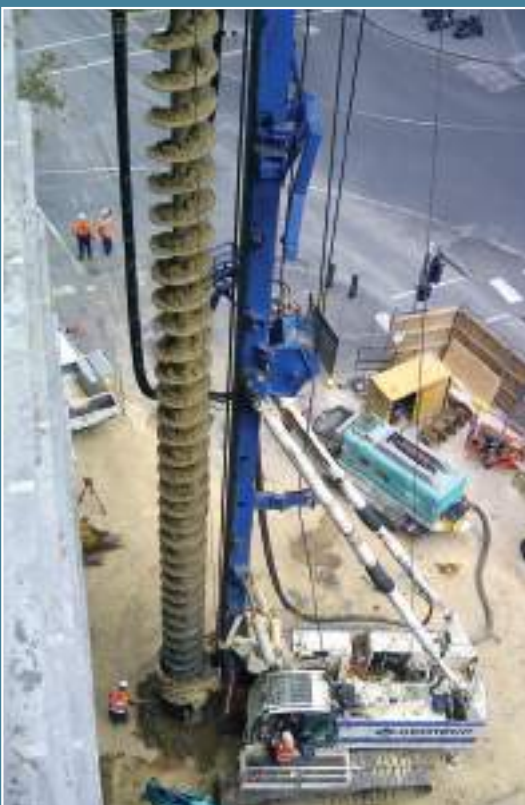
AUSTRALIA E6050 LM - CFA240 CFA Piles.
